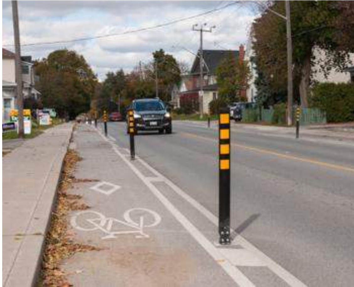
PHYSICALLY SEPARATED BIKE LANE IN ONTARIO
