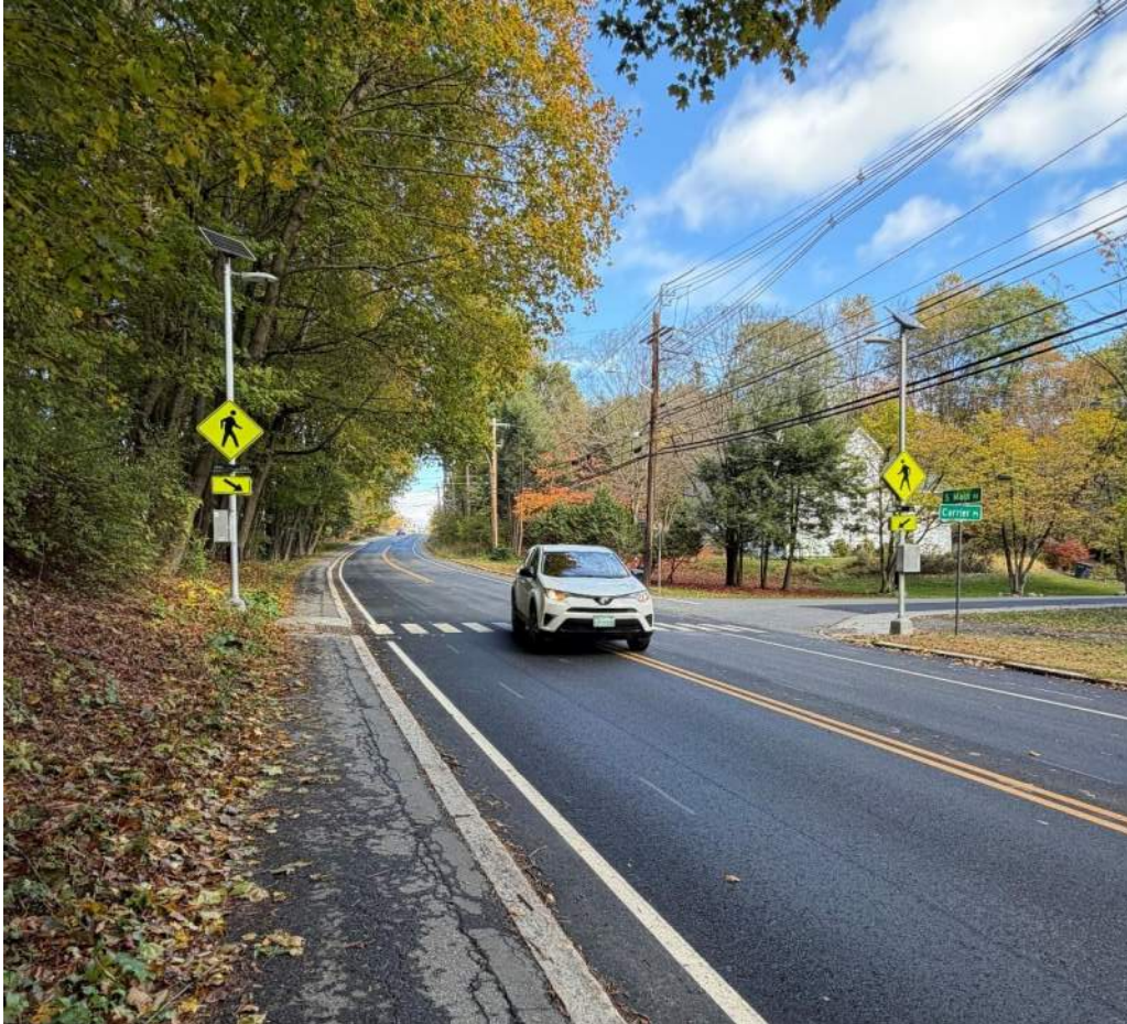
CROSSWALK WITH RRFB IN HANOVER, NH
