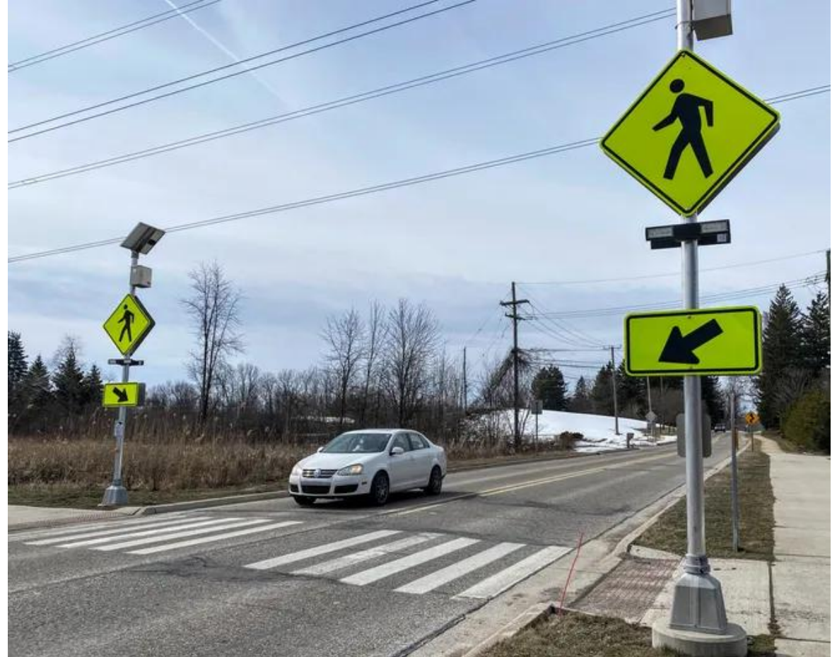
CROSSWALK WITH RRFB IN CALIFORNIA
