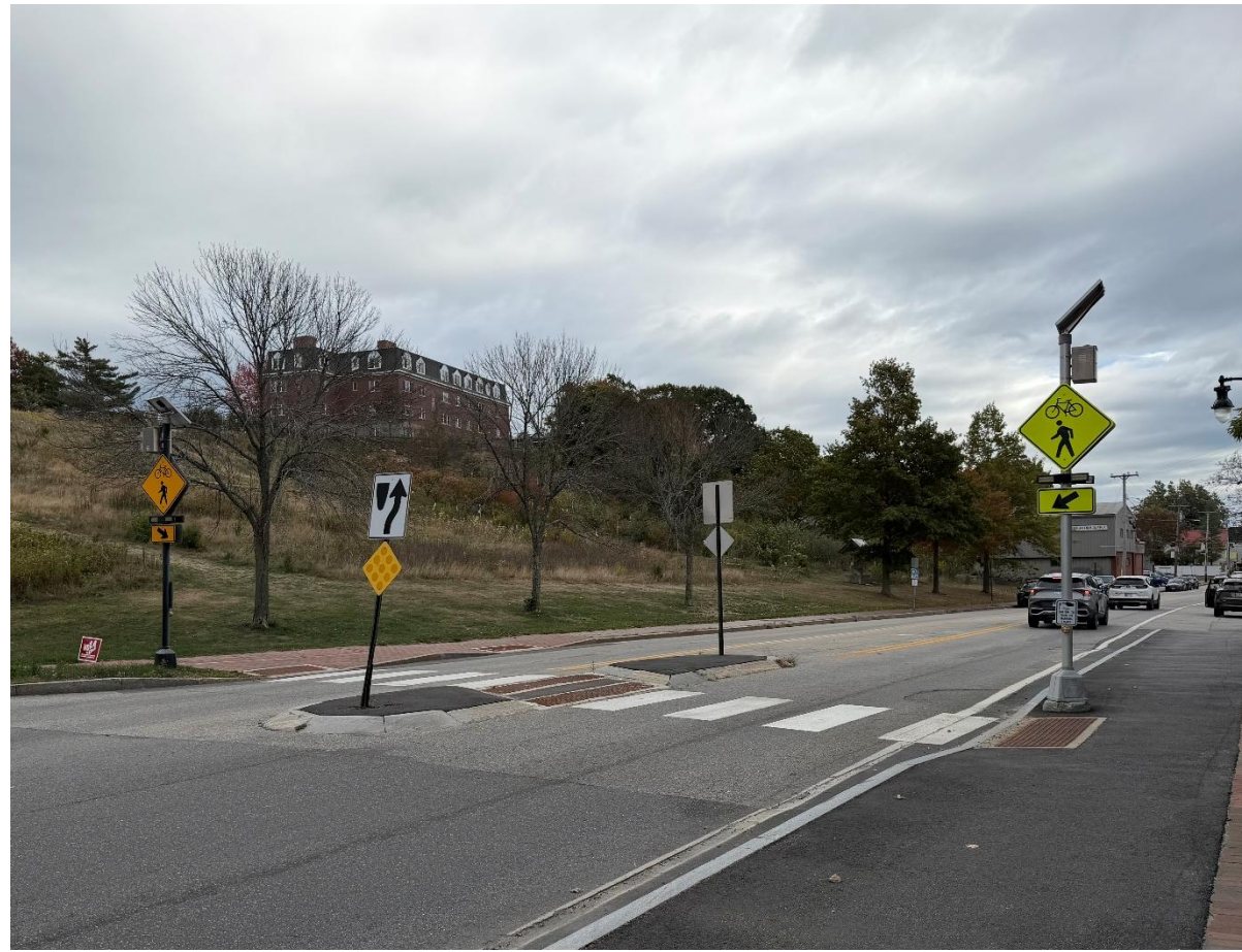
CROSSWALK WITH PEDESTRIAN REFUGE ISLAND AND RRFB IN PORTLAND, ME
