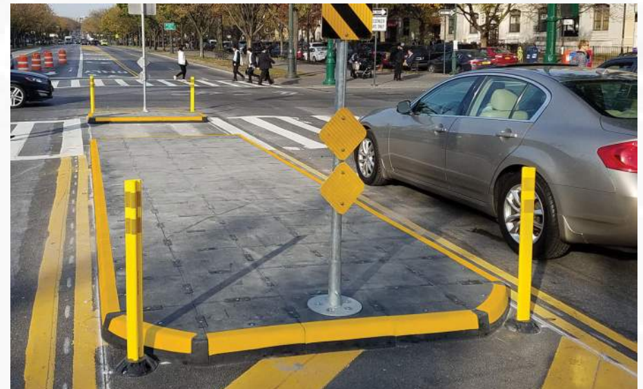
Figure 17 – Redipave Modular Median Example
