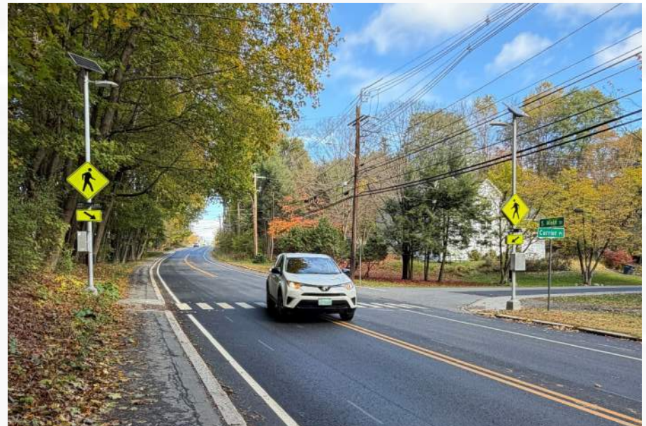
Figure 20 – Crosswalk with RRFBs Example (Hanover, NH)
