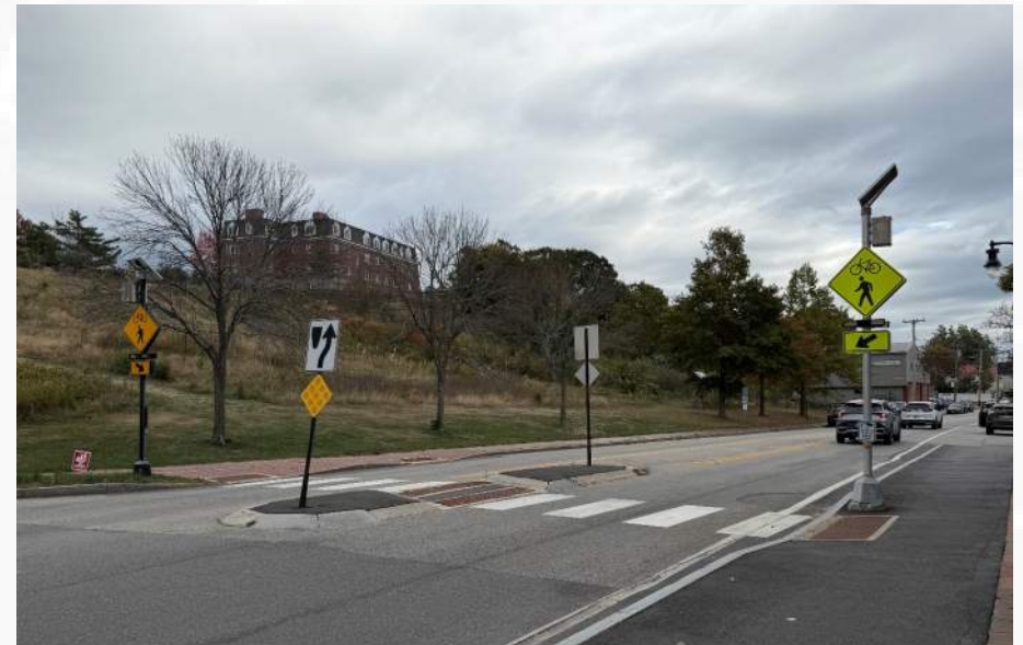
Figure 14 – Crosswalk with RRFBs and Pedestrian Refuge Island Example (Portland, ME)
