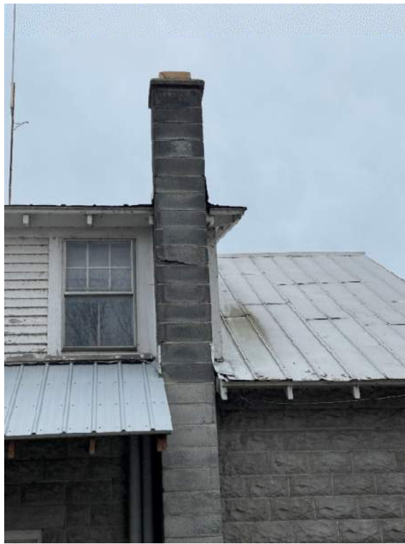
CHIMNEY DETERIORATION
