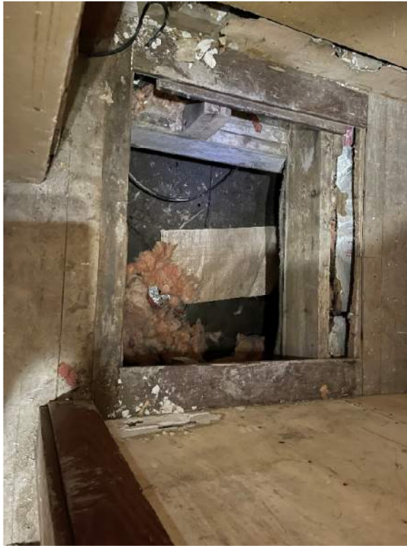
CRAWLSPACE ACCESS AT NORTH
