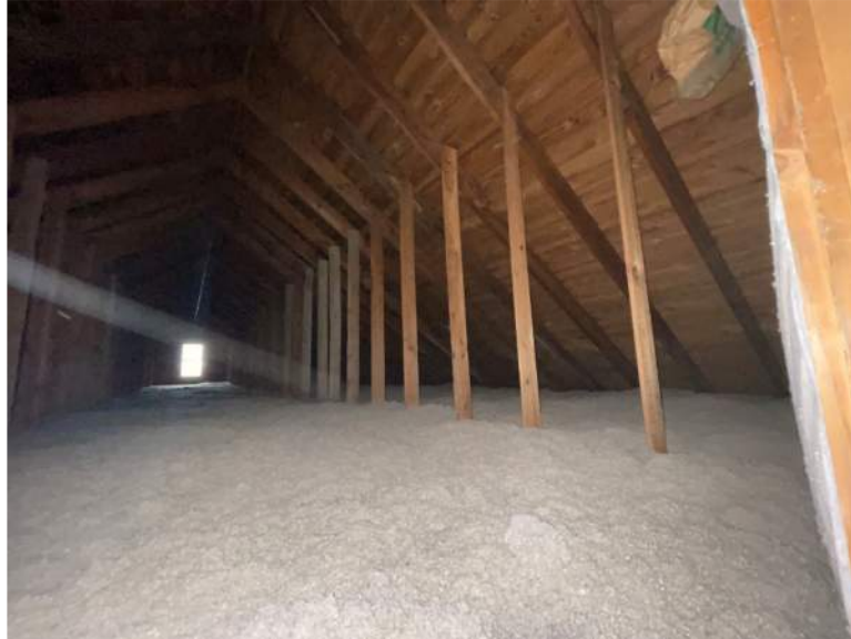
SOUTH SECTION ATTIC
