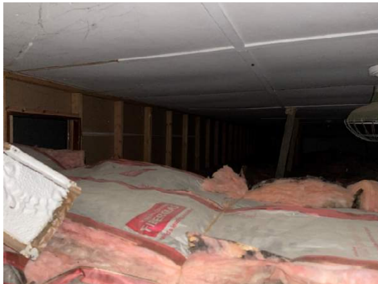
SOUTH SECTION CEILING ADDED BELOW ATTIC
