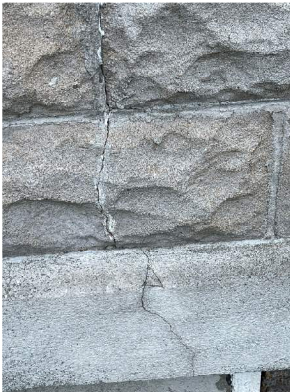
MASONRY CRACKING
