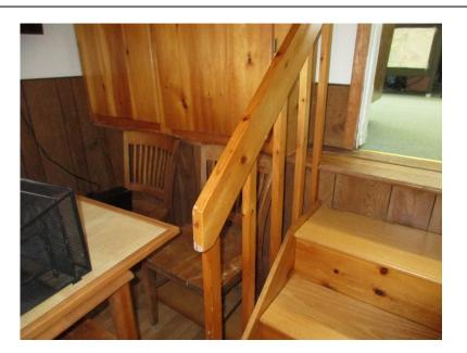
No guard railings are present at the open side of stairs. Caution should be observed to ensure safety. R312.1 Guards required.
