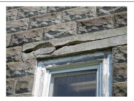
A rear leftward cinderblock as spalled away (1 block). Exposed hollow core noted is a structural concern. This cinderblock will need to be replaced as part of other exterior cinderblock work.
