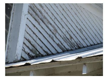
Missing siding is observed on the backside of the left dormer.
