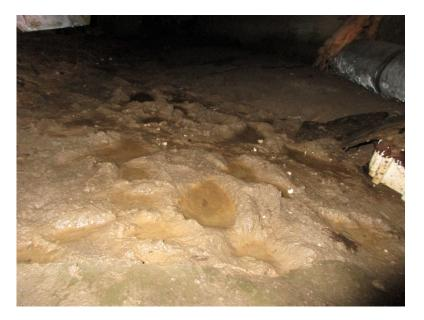
Finished areas noted in the crawlspace. Access to the original basement ceiling was not available due to wet/saturated/moldy Homasote (fiber board) now present.
