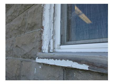
Moisture damage/soft wood is observed on the rear leftward window casing.
