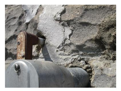
Missing caulking at all areas where cinderblocks and trim meet, including around all windows and door moldings. Without weeps (drainage in the bottom course of blocks), sealing around openings is imperative. Suggest caulking be performed to avoid water intrusion.
