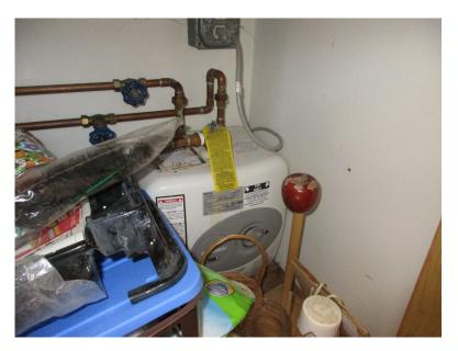
Hot water was noted at all tested plumbing fixtures indicating the electric water heater elements were functioning properly at the time of inspection. These elements are not visible or accessible to the inspector and are not specifically tested at the time of inspection. No warranty, guarantee or certification is given as to future failures.
