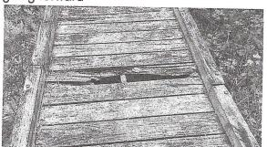
**Side Rails** need to be raised on blocks to allow water drainage and expulsion of leafy material to prevent rot
