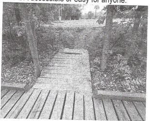
Sills were placed on top of soft soil, and are sinking into the wetland, causing the entire boardwalk to sag and become unstable.
